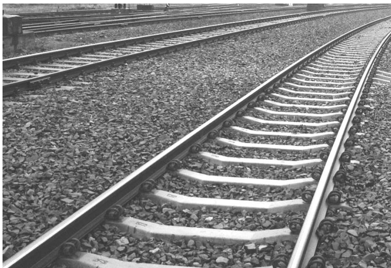
Fig. 1. Track with rail fastening type SB-3
